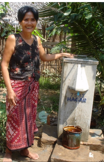
The first filter installed January 2006
